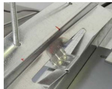
Figure 1- Note part is still attached at deemed failure.
