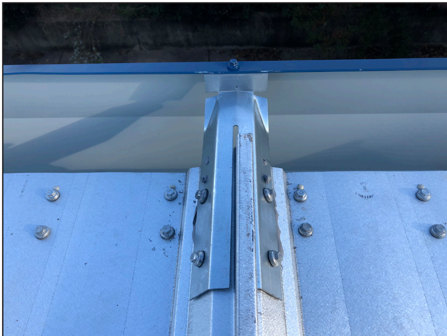
Install Gutter Support
