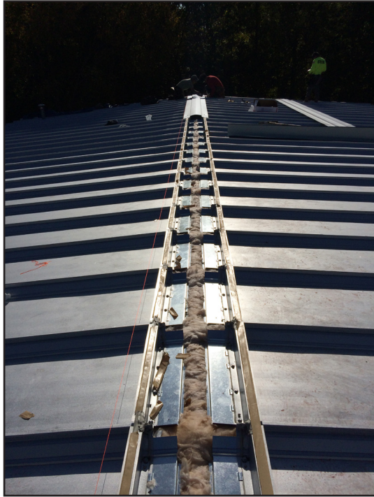
Ridge View With End Dams Installed
