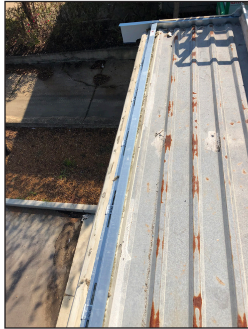
Termination with High Capacity Rake Plate - Downslope View
