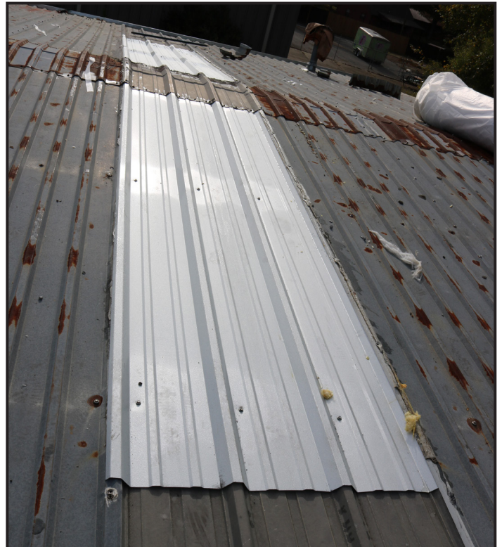
Skylight Repair with Metal Panel
