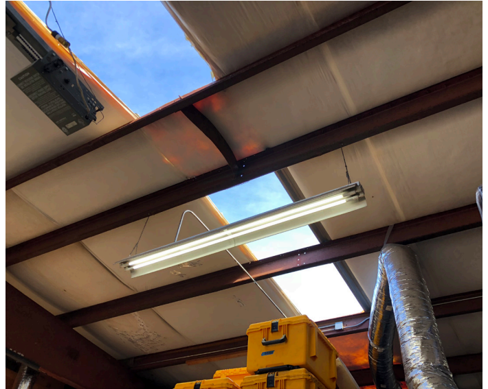
Skylight Repair with Metal Panel
