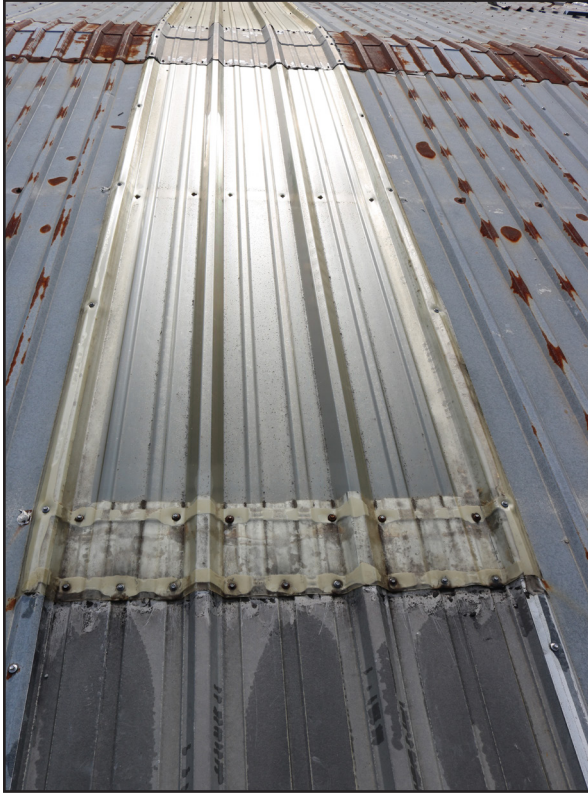
Existing Roof with Skylight
