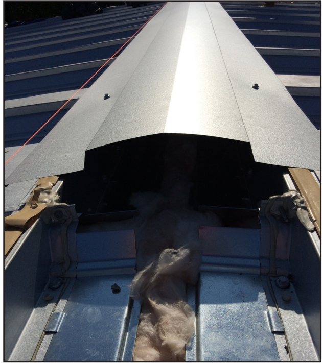
Close Up View of Ridge Cap Installation
