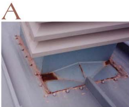
A This galvanized curb has already started rusting at the welds in less than one year.
